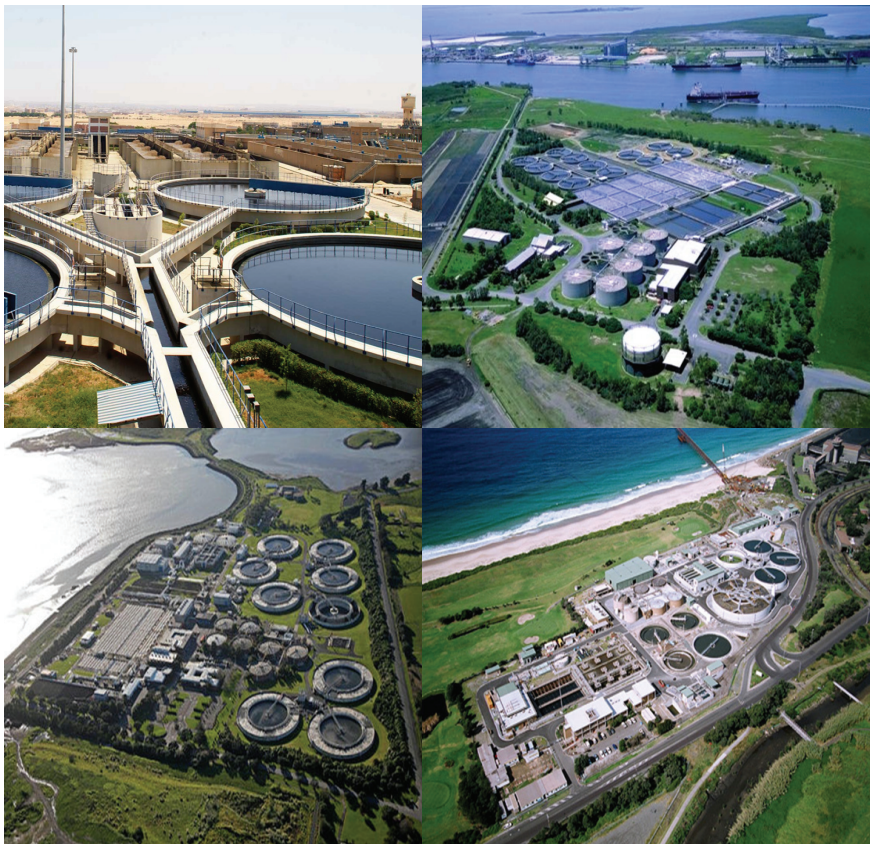
FIGURE 73 – EXAMPLES OF NEW, EFFICIENT, LIQUID WASTE INFRASTRUCTURE
