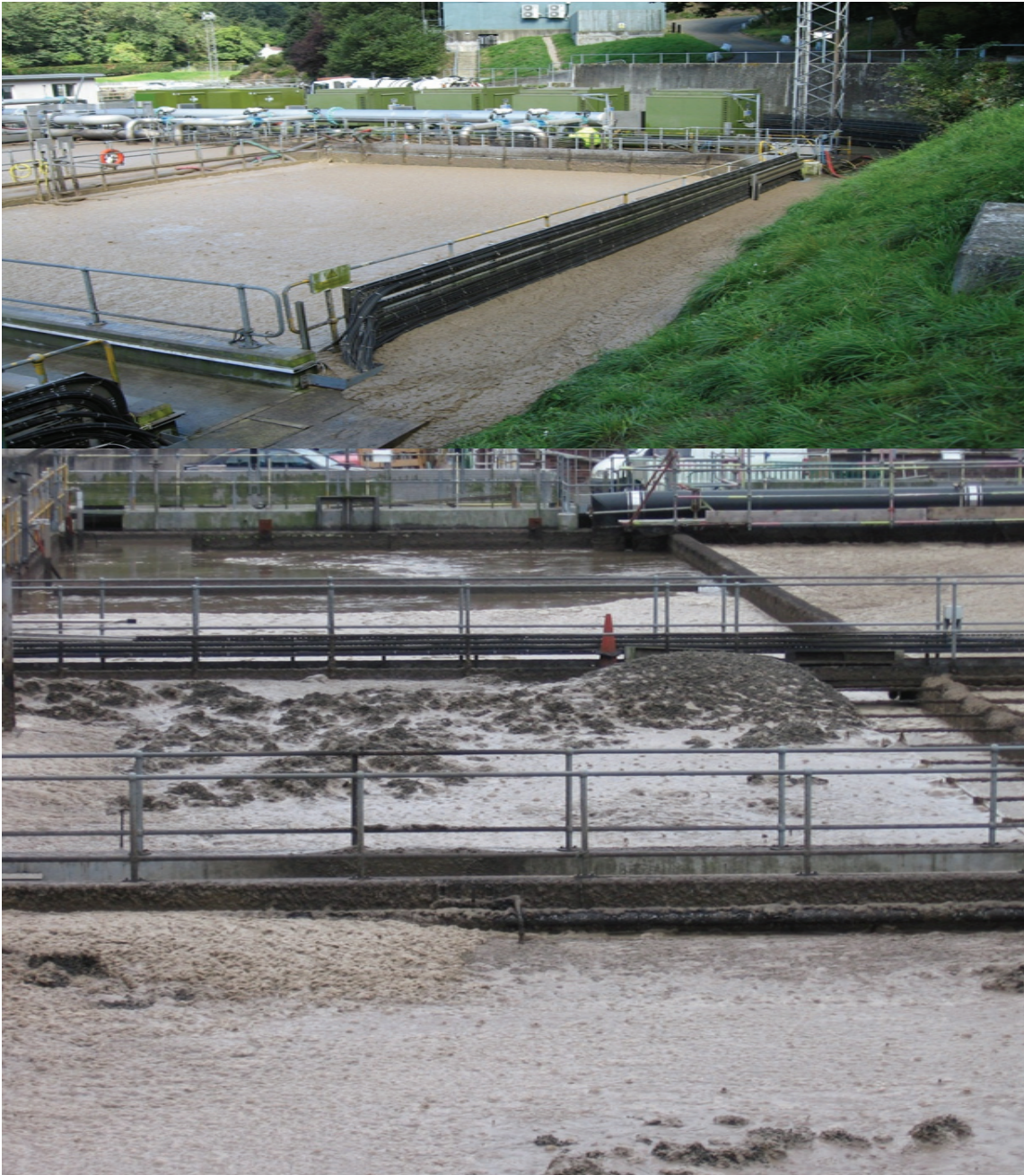
FIGURE 71 – AGEING SEWAGE TREATMENT WORKS
